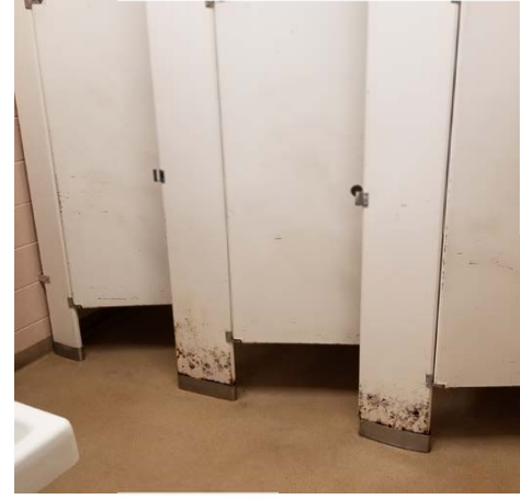
Before construction – noncompliant ADA fixtures and layout, peeling flooring, corroded stainless steel
