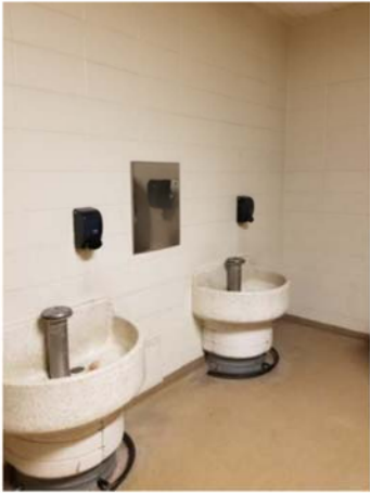
Before construction – noncompliant ADA fixtures and layout, peeling flooring, corroded stainless steel
