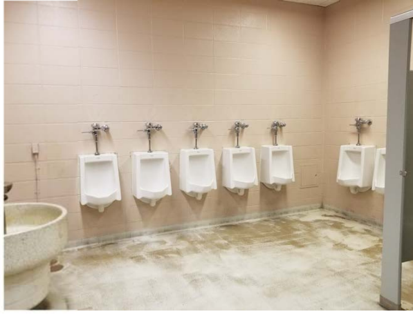
Before construction – noncompliant ADA fixtures and layout, peeling flooring, corroded stainless steel
